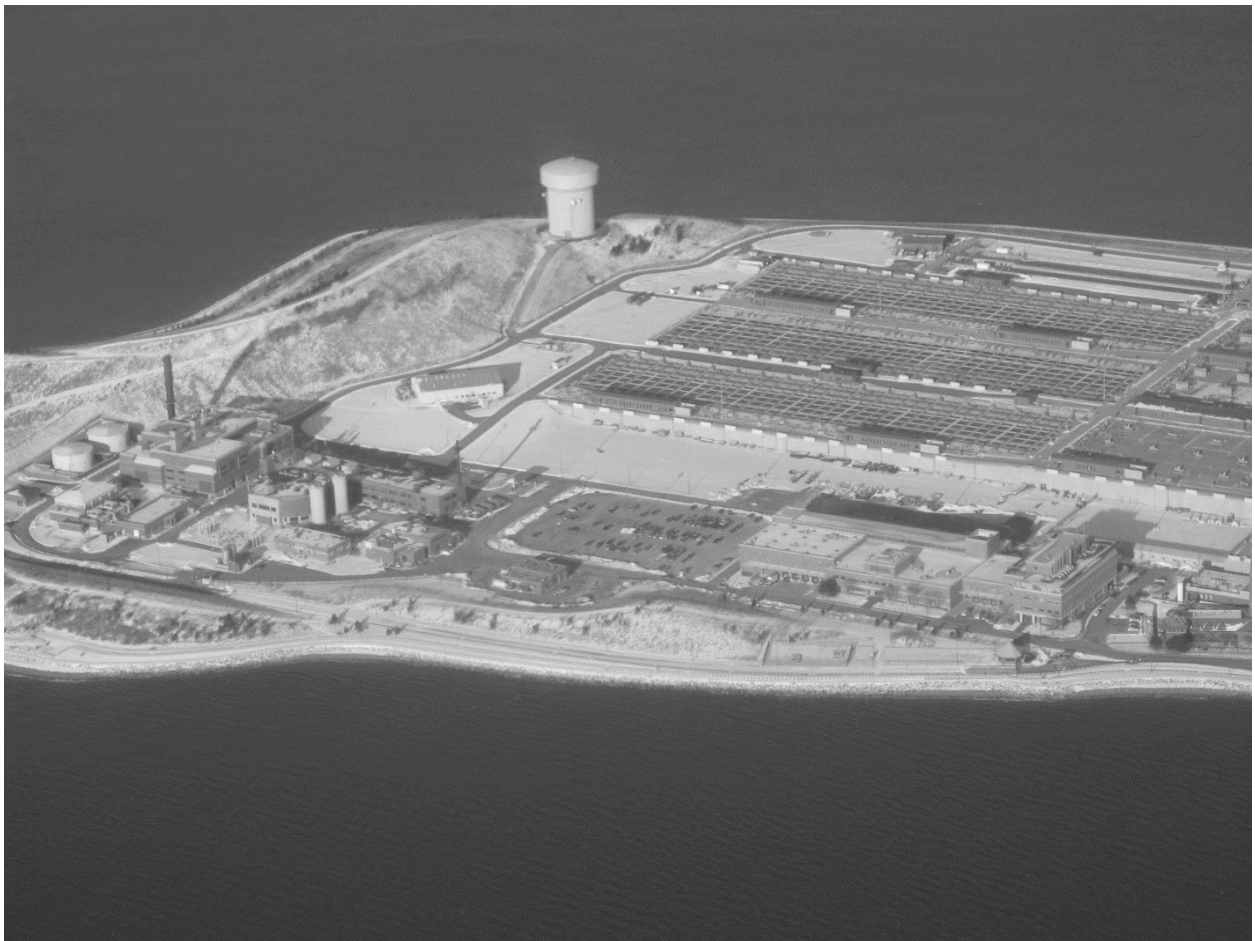
Deer Island Sewage Treatment Plant: Part of a $6 Billion Project that Helped Clean Up Boston Harbor.
