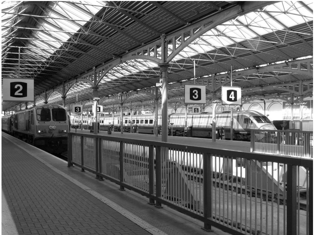
Figure 1 Dublin Train Station
