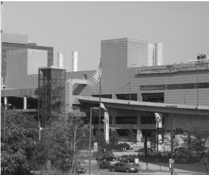
Figure 1 South Station Bus Terminal, Boston
