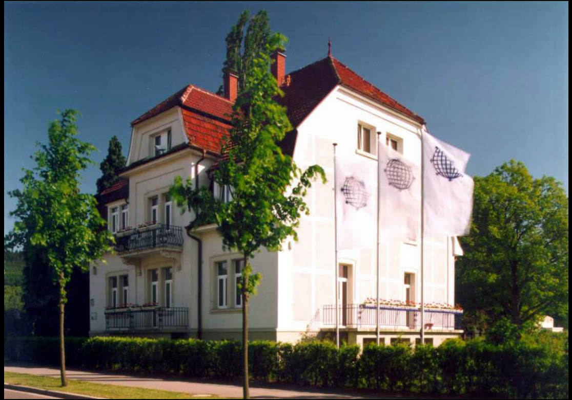
Villa Tannheim, Headquarters of the International Solar Energy Society, Freiburg, Germany (Architecture Heinzel). Photo © ISES. All rights reserved. This content is excluded from our Creative Commons license. For more information, see https://ocw.mit.edu/help/faq-fair-use/ .
