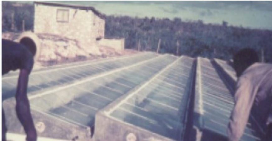
Figure 4: Fisherman of Source Phillip working on the 300m 2 solar still installation
